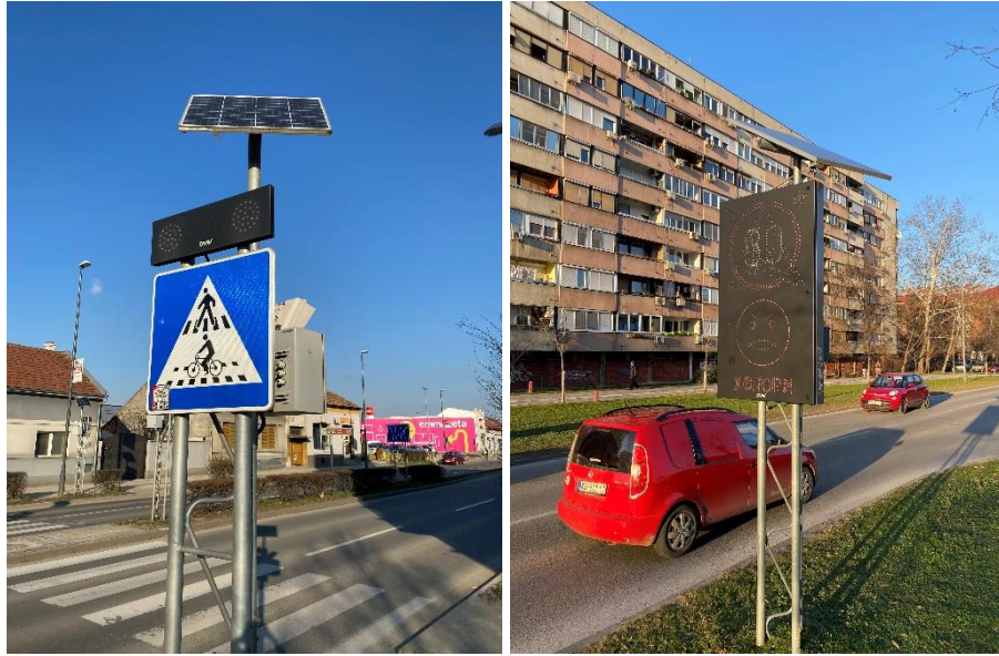
Figure 1: Solar-powered flashing traffic signs
