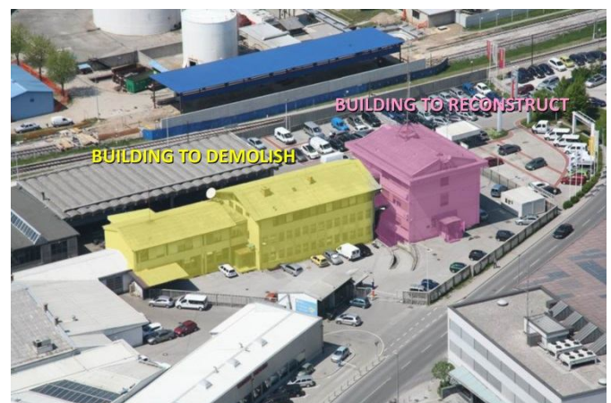
Figure 7. Existing building before reconstruction
